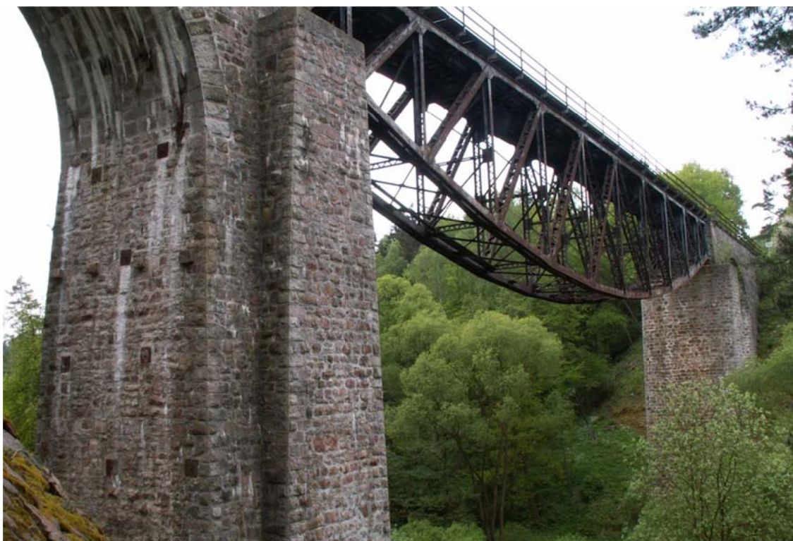
Obr. 1 Most v km 20,862 trati Rakovník – Mladotice
